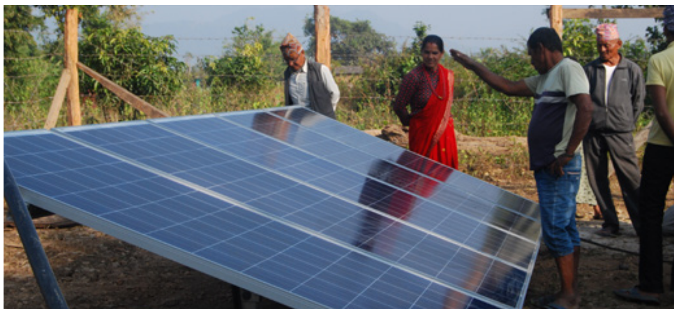
Figure 15: The installation of solar-powered irrigation system in Nepal to collect water from the river to a pond which will be used for irrigation during the dry seasons. Photo Credit: Shobha Manandhar
